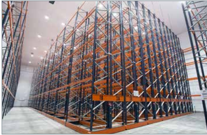
One of the chambers inside Idube's 4 700 m 2 cold store. The installation of the storage system from APC Storage Solutions SA enables Idube to store 12 000 tons of frozen product across all three chambers.
