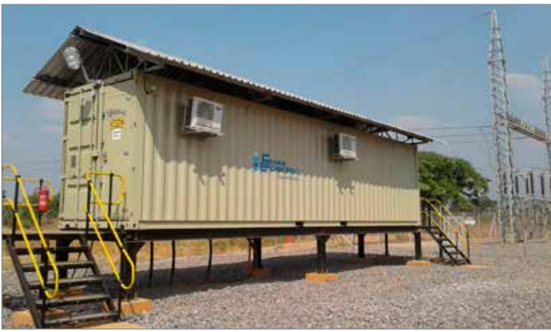
The fully withdrawable circuit breakers and voltage transformers (VTs) make the design ideal for a container, while also improving the ease of maintenance of the circuit breakers and VTs.
