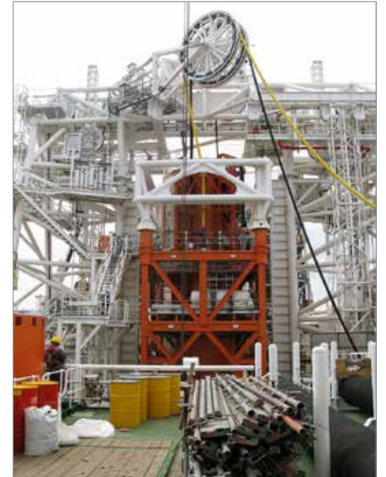
A front view of the launch and recovery system (LARS) and SBT during installation. The hydraulic ring main for the LARS comprised a central hydraulic power pack, which supplies oil through the ring main to the equipment used to launch and recover the SBT.
