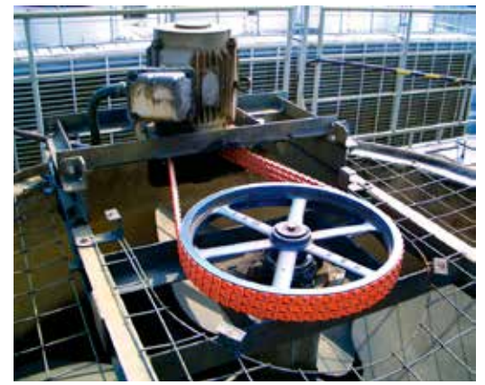
Fenner PowerTwist Drive V-belts and Quatro Plus TW heavy duty drive belts offer high performance, maximum drive efficiency and extended service life in tough conditions.
