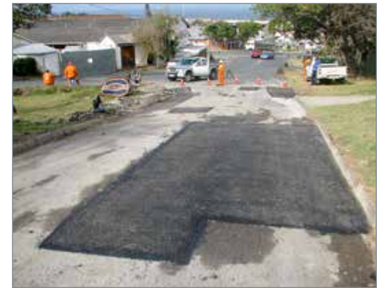
Both small and large areas can be repaired using National Asphalt's Cold Mix.
