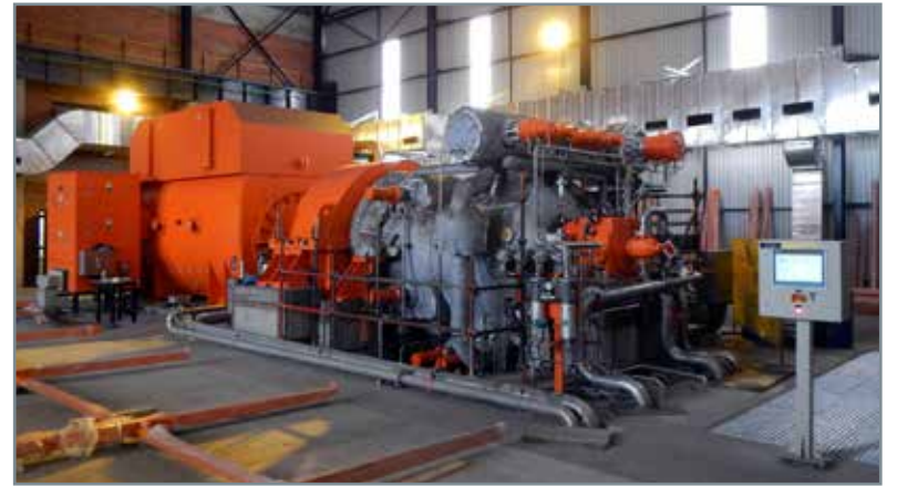
A 48 MW multi-extraction condensing steam turbo generator set, with associated auxiliary systems, used for co-generation in the pulp and paper market.
