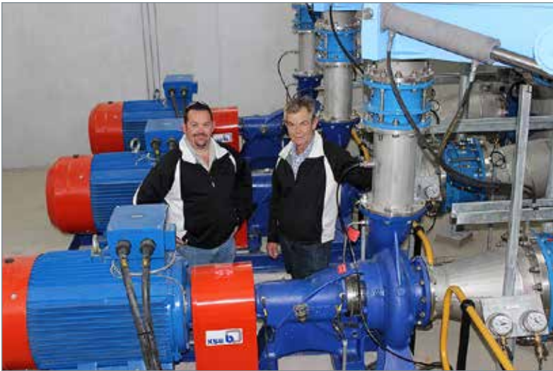
KSB Pumps and Valves' branches and dealer manager for South Africa, Francois Naude with regional sales manager (Sub-Saharan Africa), David Jones, at the Leliefontein pump and turbine station (PaT).
