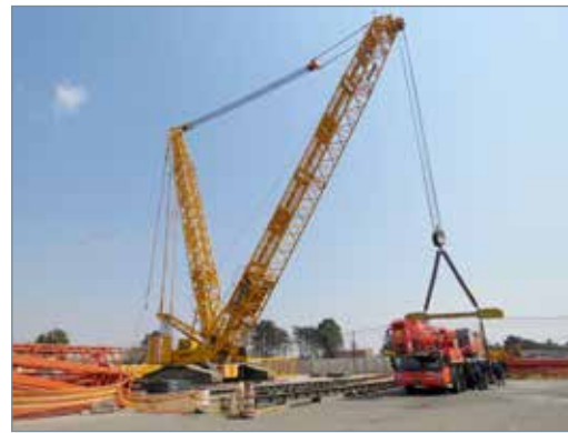
The Johnson Crane Hire 600 ton lattice boom crawler crane towering over the 275 tonner.
