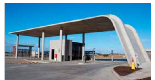
The arched and sloping walls were 10 m x 7 m, while the actual feature brow was 25 m long.
