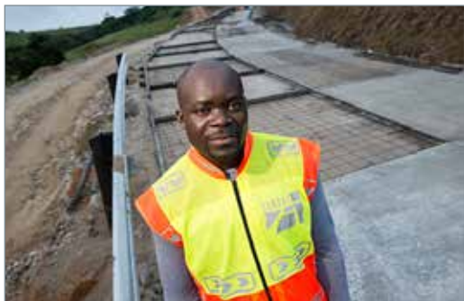
Emmanuel Sisanda's company First Building Construction has helped to create much needed jobs in the Msikaba area.
