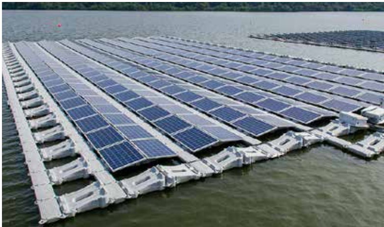
A floating ABB PV panel platform in Singapore. Source: greentechmedia.com, technology.ihs.com
