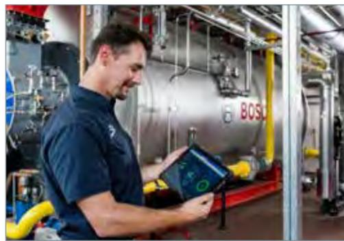
an energy management system. Since 2017, the company has also been using the digital efficiency assistant MEC Optimize from Bosch, which now enables predictive maintenance.
