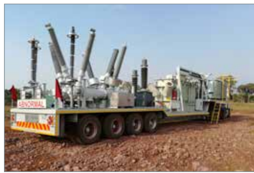
Preparations underway to start with the scope of work on site.
