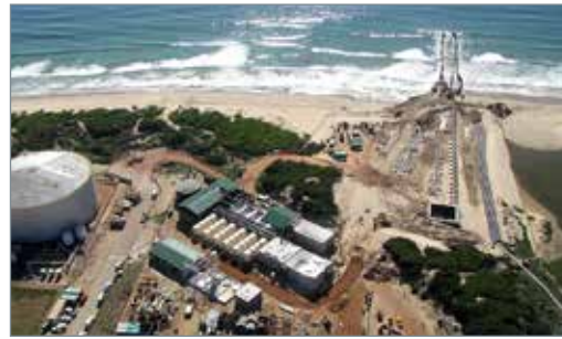
South Africa's largest desalination project - 15 Ml/day Mossel Bay plant, under construction in 2010. Photo credit Royal HaskoningDHV.
