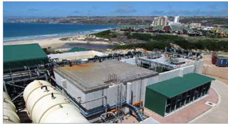
15Ml/day plant at Mossel Bay.
