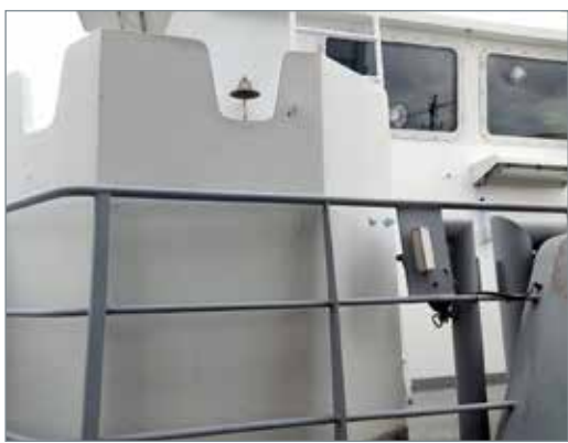
Part of the ballistic protection on the starboard wheelhouse.
