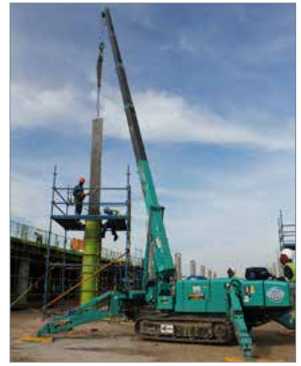
The Maeda crawler crane assisting with the build at Table Bay Mall.
