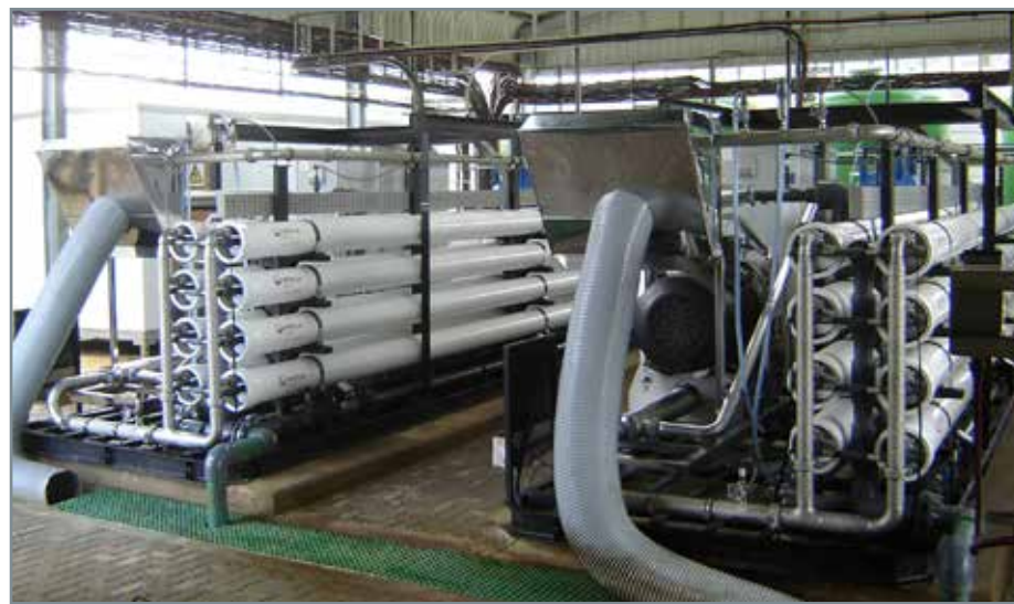
Reverse Osmosis (RO) units at Knysna desalination plant. Credit: Veolia Water.
