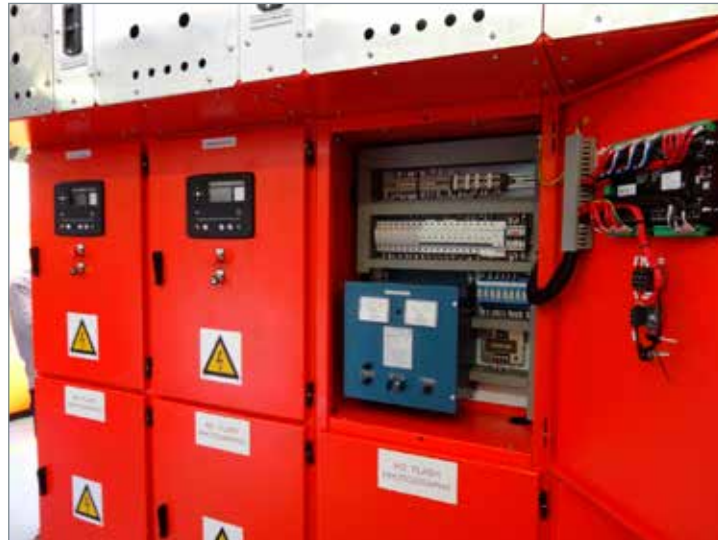
Q Range Generator Control System.
