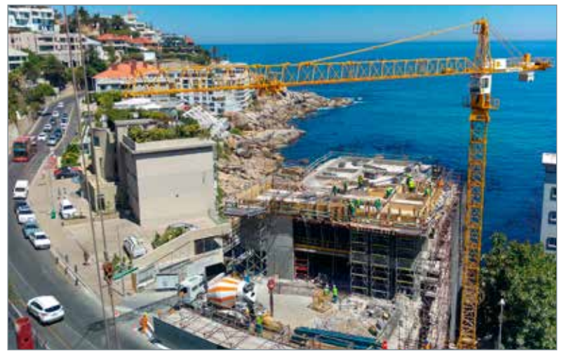
Construction work on the Aurum Development.
