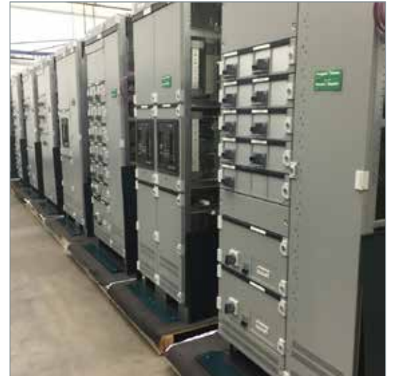
Sivacon - 58 low voltage switchboard.
