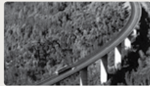
Hugo's River Viaduct
