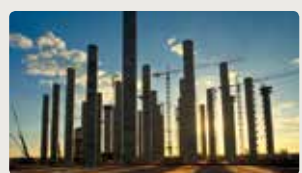
Medupi Power Station
