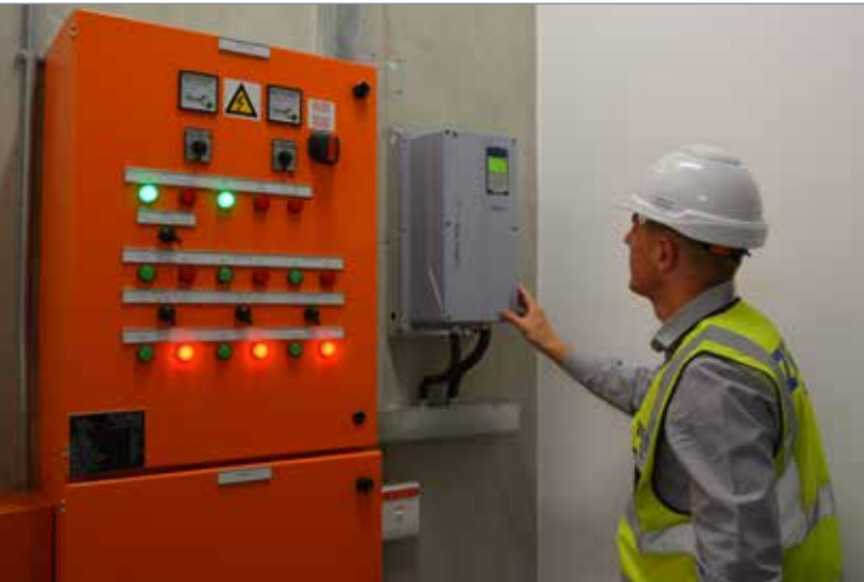
WEG CFW701 IP55 variable speed drives and control panels for the air handling units located on each floor of the PwC Tower.
