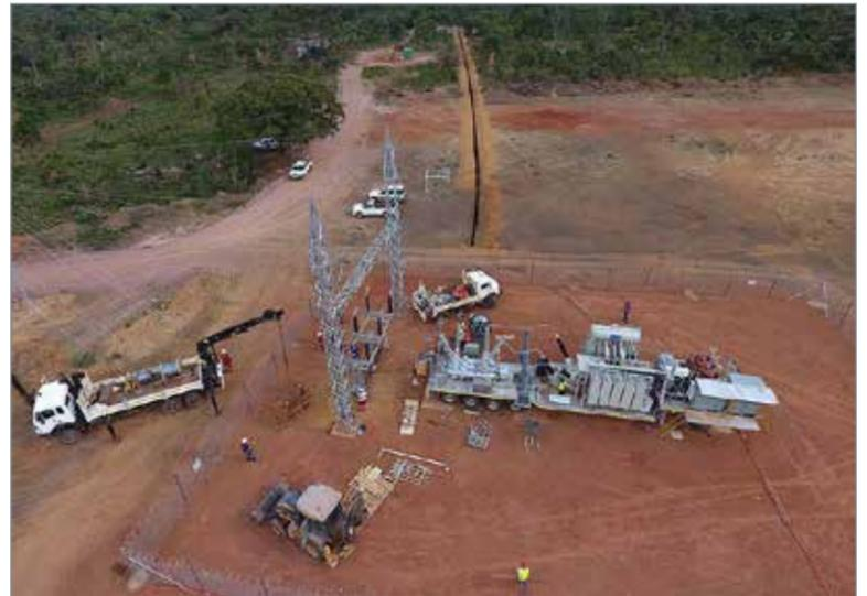
The Zest Energy mobile substation in position on site, connected to the SNEL electrical network. The photograph shows preparations for hot commissioning and energising in progress.
