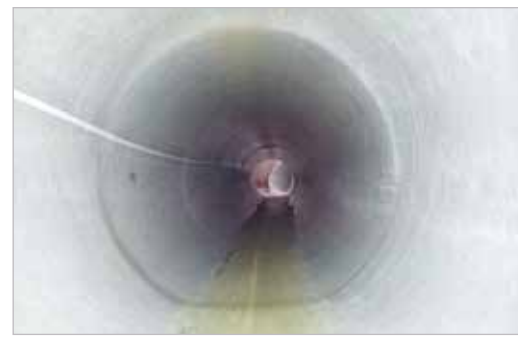
View of a rehabilitated pipeline.
