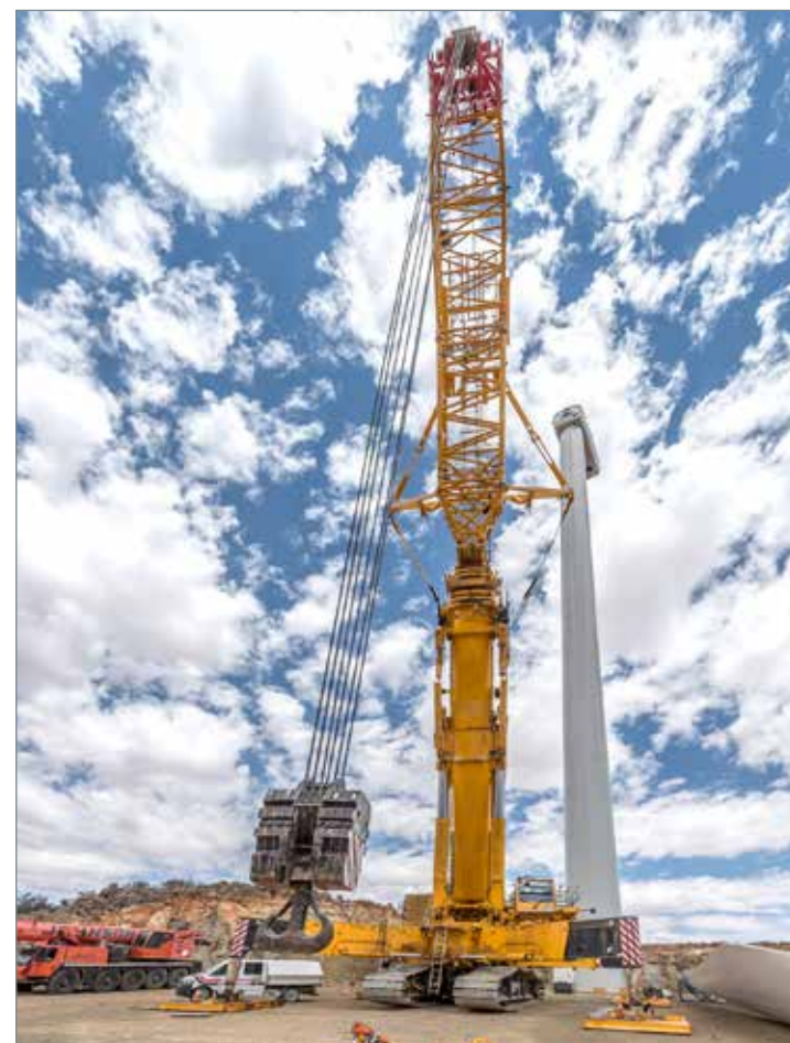
LTR 11200 undertaking the main installation lifts at De Aar wind farm.
