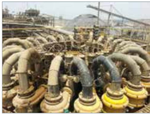
24 DeZurik KGC knife gate valves installed on a cyclone cluster.
