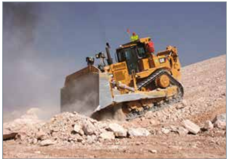
Burma Plant Hire is an active player in landfill and rehabilitation work.
