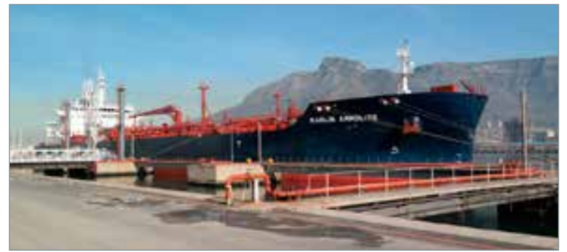
The first liquid bulk vessel discharged product at the Borgan Cape Terminal at the Port of Cape Town during the first week of July 2017.
