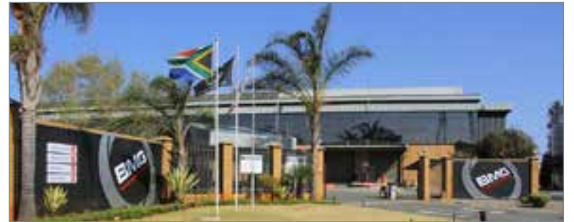
BMG marked the official opening of the recently upgraded ‘BMG World’ distribution and engineering facility in Johannesburg, by hosting a two day expo in September for suppliers, customers, the press and staff.
