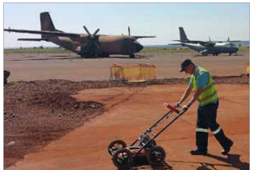
Bosch Munitech USL facility - GPR Scan at an airforce base. Its underground services location facility provides reliable information on buried infrastructure services.
