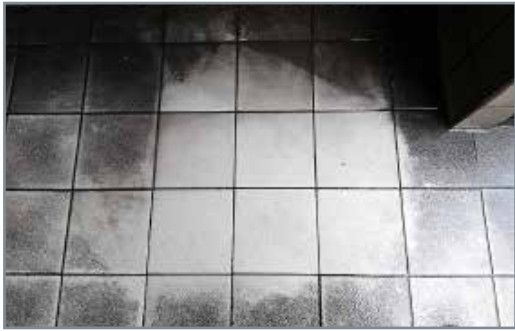
Heavily contaminated floor treated with Wipe Out.
