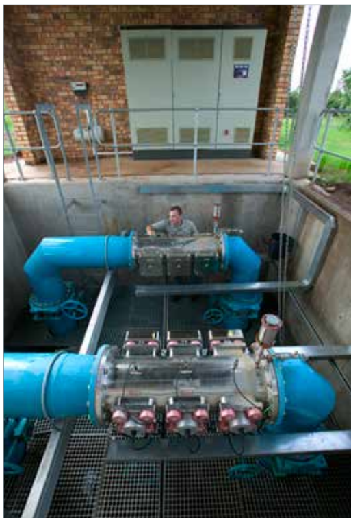
Municipal atg UV system in South Africa.
