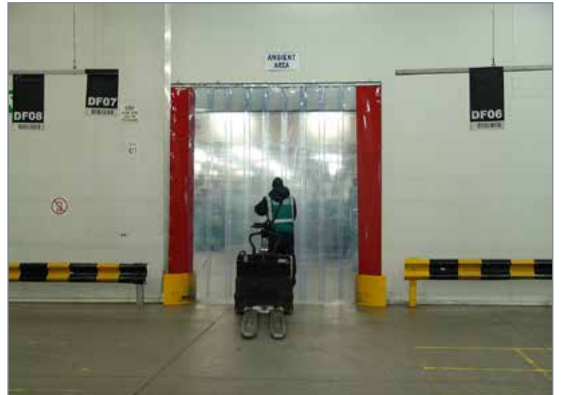
Apex Strip Curtains allow the unhindered and safe passage of people and forklift trucks.
