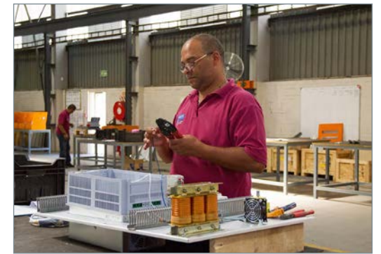
Assembly of a variable frequency drive panel (VFD) under at Zest WEG Group's facility in Cape Town.
