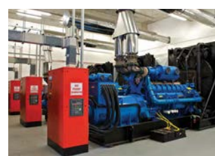
Six 2 000 kVA open type synchronising generator sets
