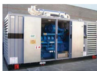
Containerised 1 250 kVA generator set
