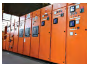
SC100 Motor Control Centre
