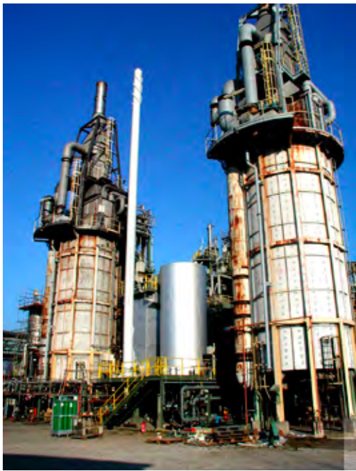
The new heater plant impresses with modern three-pass technology, boasting only a very small footprint despite the same high power output.
