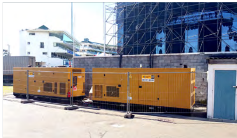
Barloworld Power generators supplied power to the KDay 2015 music festival at Newlands cricket ground on 28 February.
