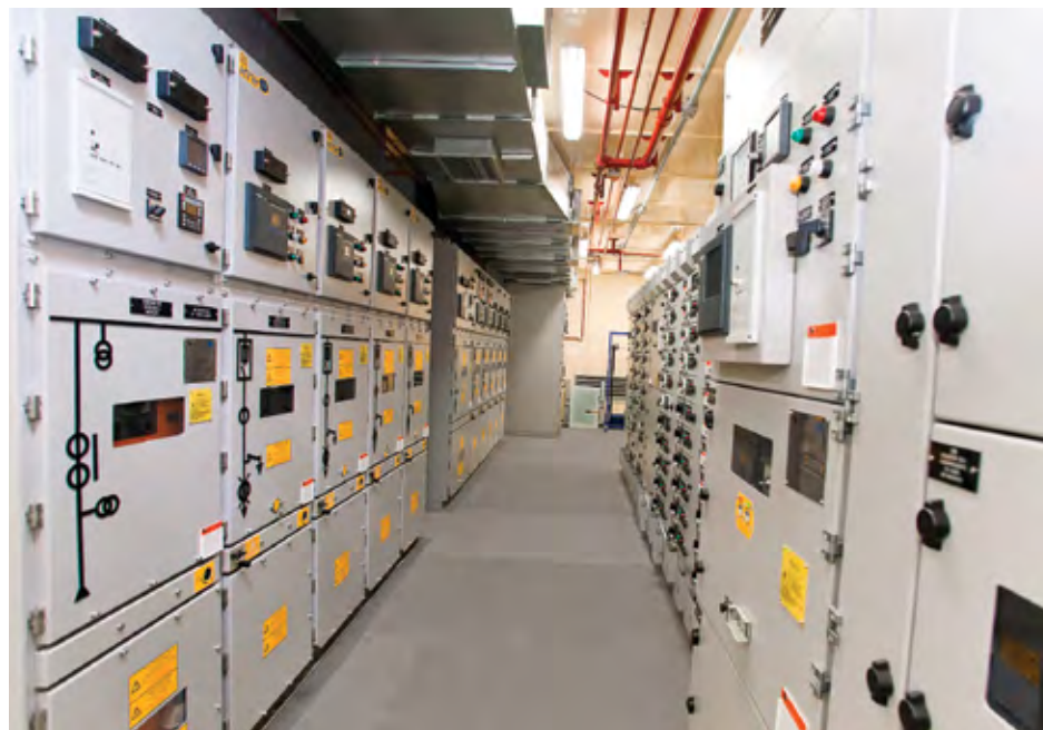
LV and MV Switchboards inside "E" House
