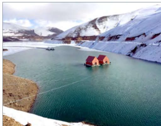
Pontoons on tailings dam at Sungun Mine.
