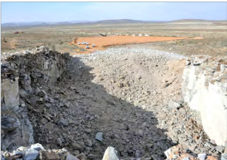
NMC Civils has started work on 80 kms of road infrastructure for the SKA site.
