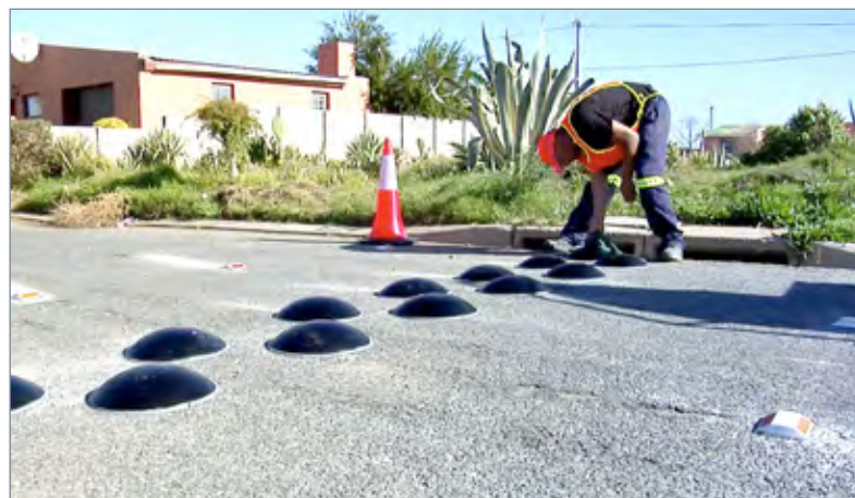
By training youth and women to install the system, Dura Bump supports municipal EPW programmes.
