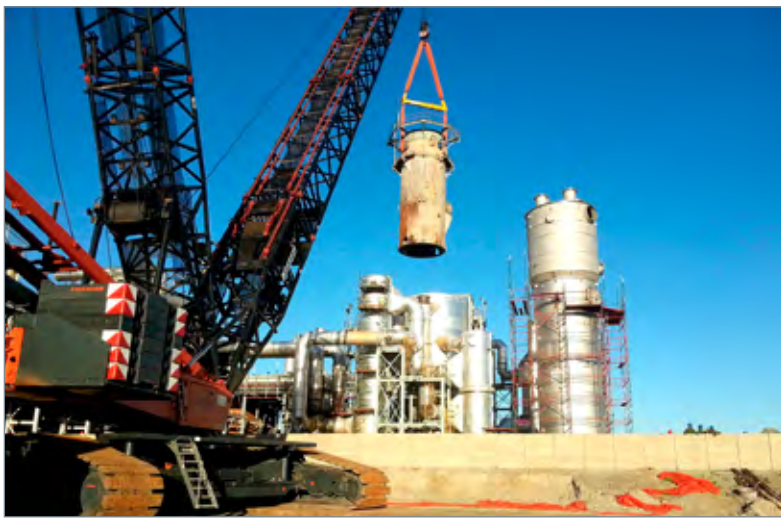
This Johnson Crane Hire 750 t Liebherr crawler is configured with super lift for a lifting project at Waterval Smelter.
