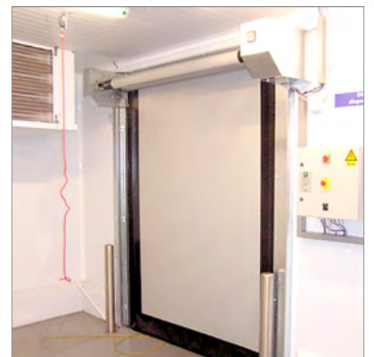
The Albany HS9010PFR is a high speed door specifically designed for freezer environments.
