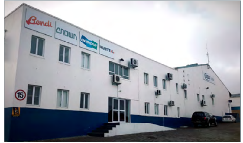
Goscor's new Cape Town premises.
