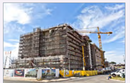
Murray & Roberts Western Cape is building the Melomed Hospital in Tokai for the Melomed Group.
