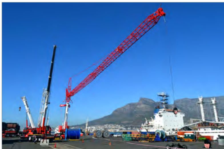
Summit Cranes new 400 ton crane's longer reach and heavier lifting capacity offers more versatility on site.
