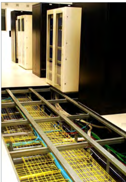
The Bergvik ISO floor panels can be removed without the floor shifting.
