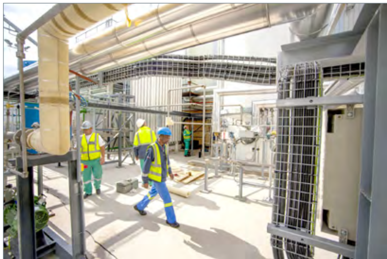
Air Products South Africa achieved its goal of 'Every one home safely, every day' in the recently completed construction and commissioning of its R300m air separation unit in the Coega IDZ.
