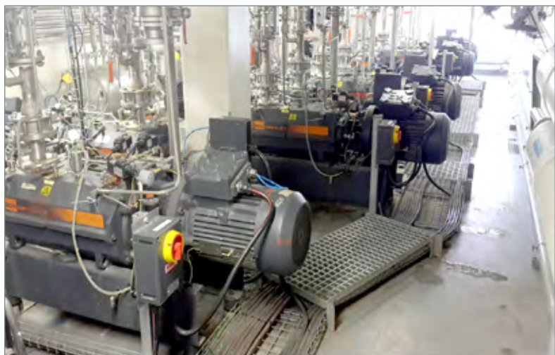
Installation of twelve Busch Cobra NT0400 Atex rotary screw vacuum pumps with PLC control panels.
