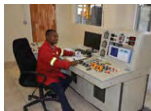
100 MVA 132 kV Testing Bay
