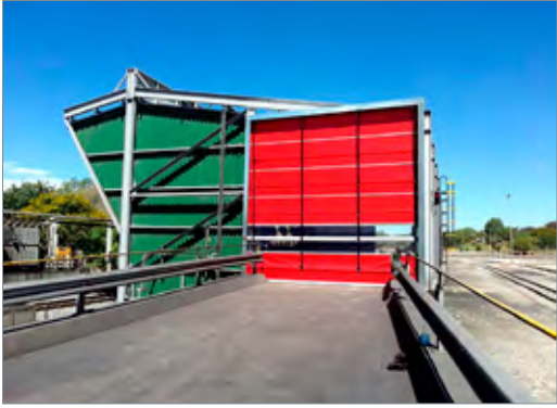
High speed doors, unlike the conventional roller shutter door, are quick and easy to open, and contribute significantly to improved productivity.
