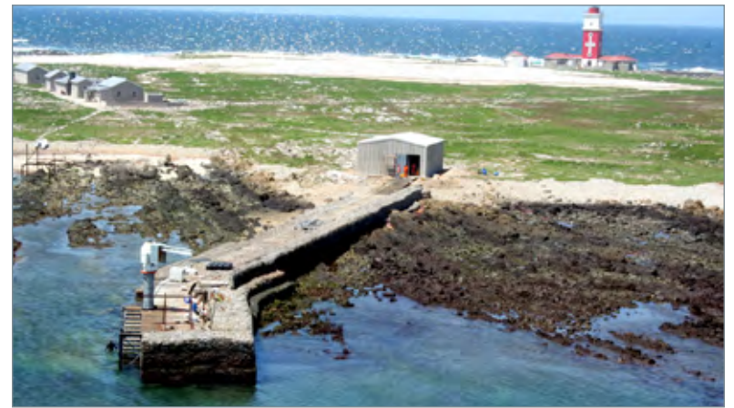
Jib crane, jetty and boathouse.
