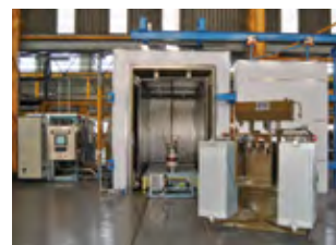
Newly Commissioned Vacuum Drying Oven
