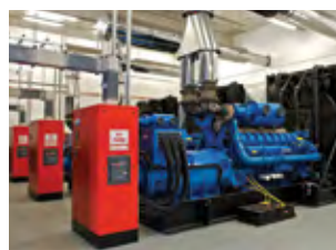
Six 2 000 kVA open type synchronising generator sets
