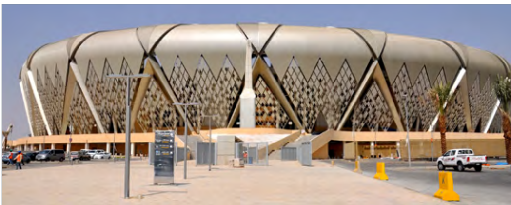
Saudi Arabia's King Abdullah Football Stadium with one of the three totems clad with vitreous enamel steel panels supplied by Vitrex.
