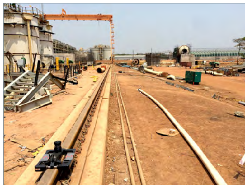
Rail Q being done at First Quantum Mine Kalumbile, Zambia.
