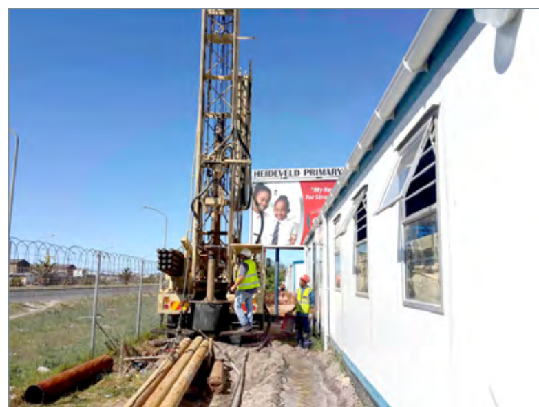
Drilling a borehole in a confined space was one of the challenges SRK overcame in this project.
