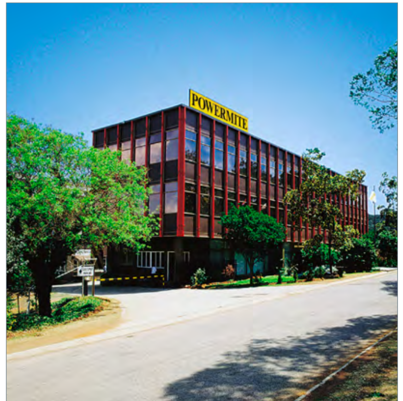
Powermite head office in Roodepoort, Johannesburg.
