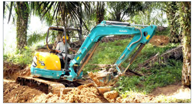
The zero boom-swing and zero tail-swing features of the mini excavator are integral in changing the dynamics of construction sites.
