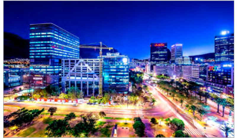
Murray & Roberts Western Cape was responsible for the refurbishment of the two tower Merriman Square, also known as The Towers, in the Central Business District of Cape Town.
