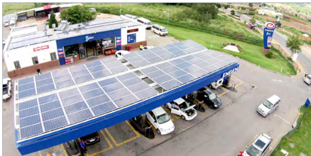
All Africa Convenience Centre in Alexandra is currently being used as a test site for solar power installations.
