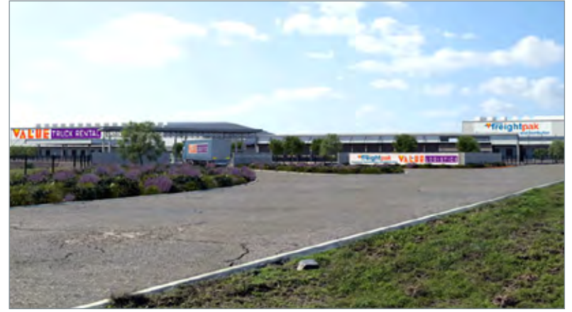
New state-of-the-art warehouse facility in Joostenbergvlakte, Western Cape. Opened in January 2015.
