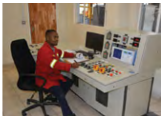
100 MVA 132 kV Testing Bay
