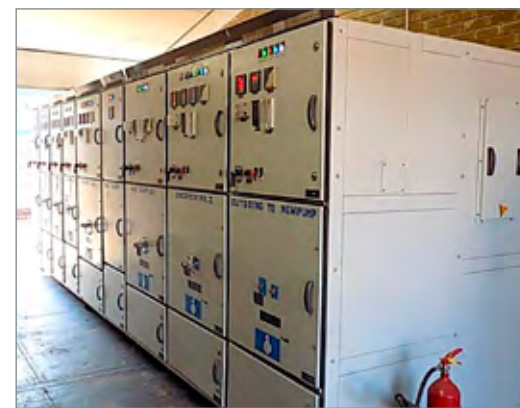
An 11kVA incomer from Eskom at Chileka pump station.
