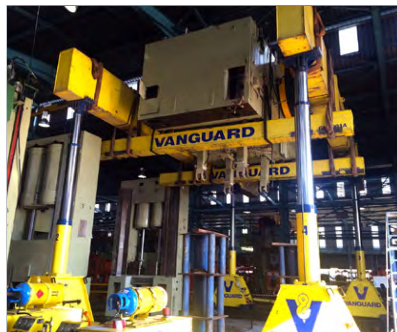
Because they came in one piece, the presses were the heaviest components.
