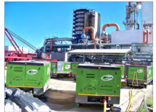
Understanding the requirements of the hiring of portable compressors and generators, Rand-Air was able to accommodate the need for the units that contributed to the overall success of the shutdown.
