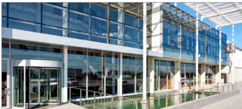
This beautifully detailed reception area, with an exposed steel supporting structure to the glass fronted with ponds and décor that turns this otherwise good industrial project into an absolute winner.
