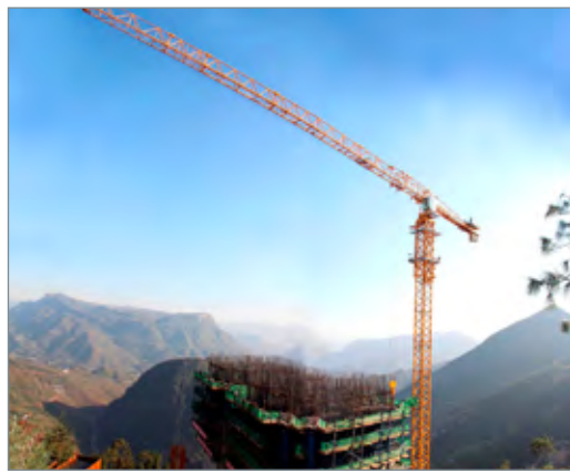
Productivity of a tower crane could also be compromised if it is not correctly configured as it would then not operate optimally. Here a Potain MCT 370 is being used to handle materials on a dam construction project.
