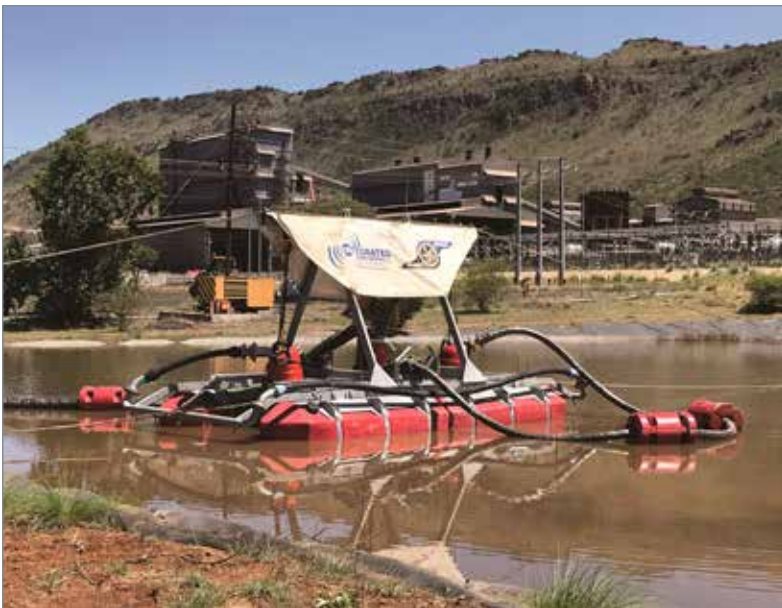
The SlurrySucker cleaning a tailings dam at a chrome mine.
