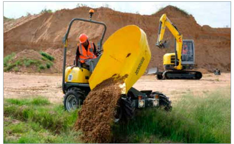
A Wacker Neuson 1601 dumper at work.
