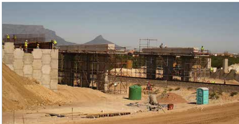
The first road-over-rail bridge built here in 2013. The second bridge now commissioned runs parallel to the first bridge built.
