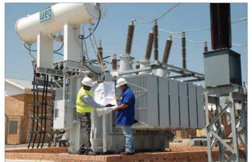
A 20MVA 132kV WEG power transformer installed on the Eskom grid.
