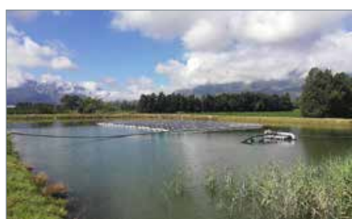
The floating solar PV system installed on a dam at Marlenique helps to prevent evaporation and saves land for agricultural use.
