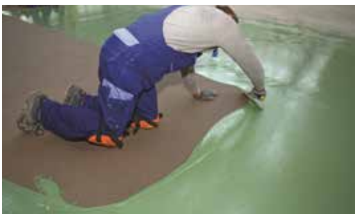
The Mapefloor system being applied.
