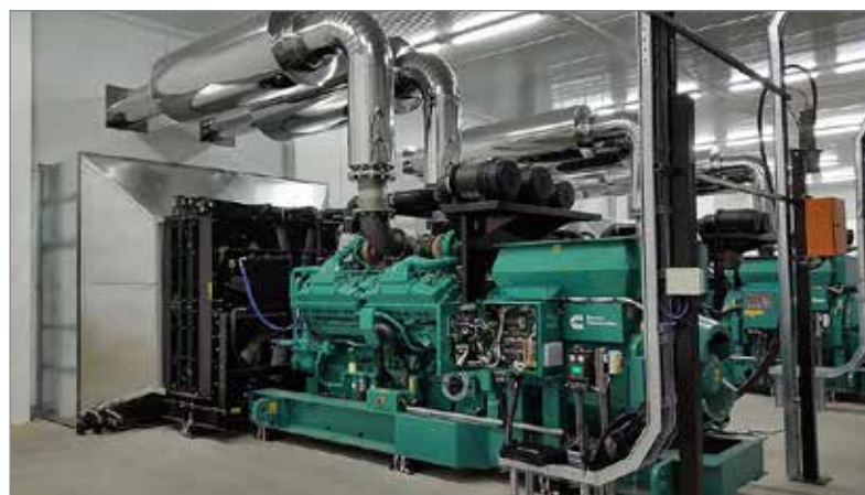
An example of a standby power generation solution from Cummins.
