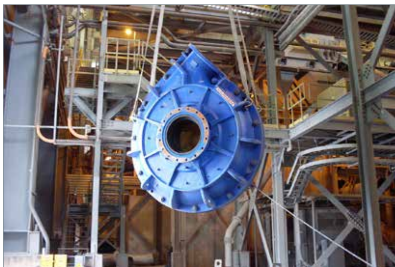
Warman MCR with reverse rotation during installation.
