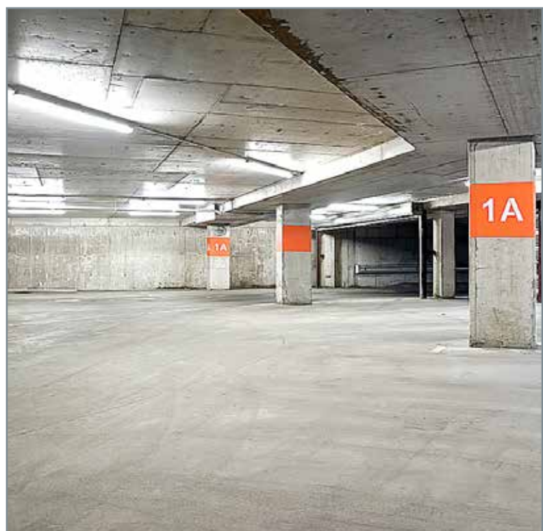
Concrete floors for success depend on a full understanding of the product used as well as all the phases of the laying process, says The Concrete Institute MD, Bryan Perrie.
