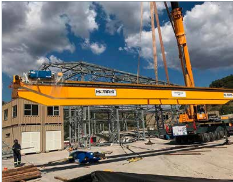
Image shows a recent installation of a 10 ton, 16.5m span, 7m height of lift, Double Girder ABUS EOT crane at a platinum mine located in Lydenburg, to be utilised in a central mine workshop building. Project completion date estimated end of July 2019.
