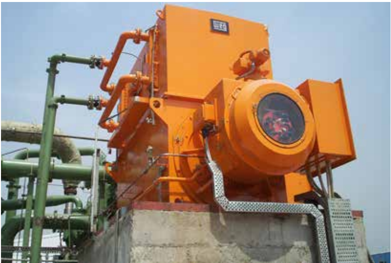
WEG wound rotor induction motor installed on site.
