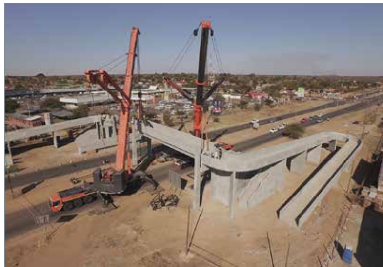
Upfront engineering on a tandem bridge lift by Johnson Crane Hire saw the lifting project successfully completed.
