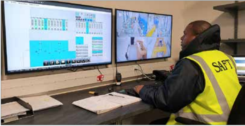
Fully computerised monitoring systems control all aspects of product through the facility.
