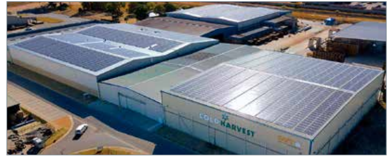
Paarl Cold Harvest solar installation.
