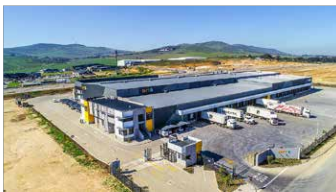
Aerial view of the new SAFT Atlantic Hills cold storage facility.
