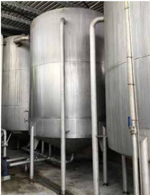
Processing tanks in LDX 2101 stainless steel supplied by NDE to a local fishing industry customer.
