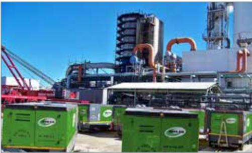
Rand-Air supplies temporary compressed air and power to oil refinery shutdowns.
