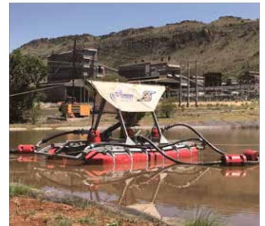
The SlurrySucker cleaning a tailings dam at a chrome mine.
