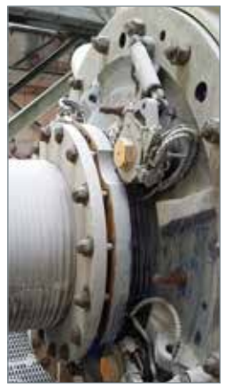
Adjustment mechanism reduces throatbush wear.
