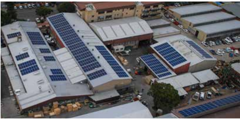
684 Photovoltaic (PV) solar panels were installed at Multotec providing almost 20% of the daily electricity demand.
