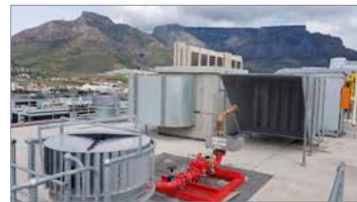
Fire protection for heli-pad on the roof top of Christiaan Barnard Hospital.
