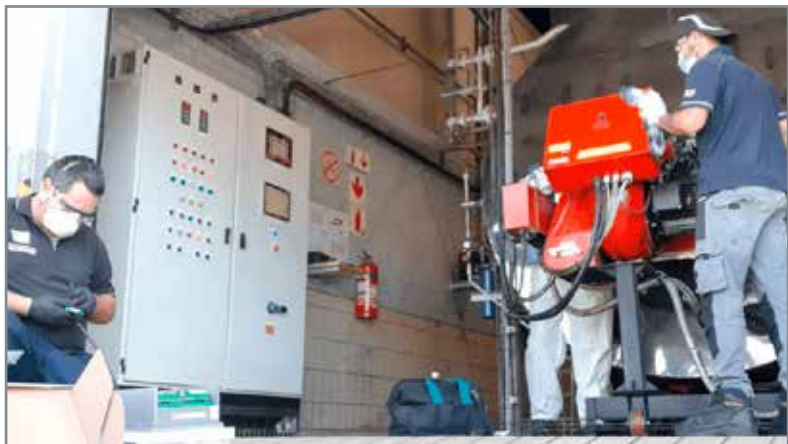
A number of service engineers in the field showing their commitment to the global fight against the Corona virus. They are remotely monitoring client's boilers and are able to react timeously to ensure continuity of essential services.
