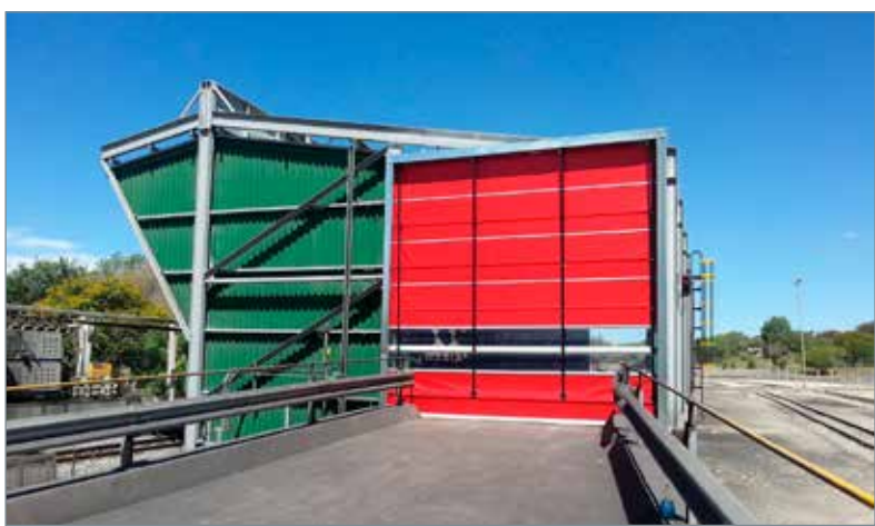
The Apex range of high speed doors incorporates a counterweighted balancing system.
