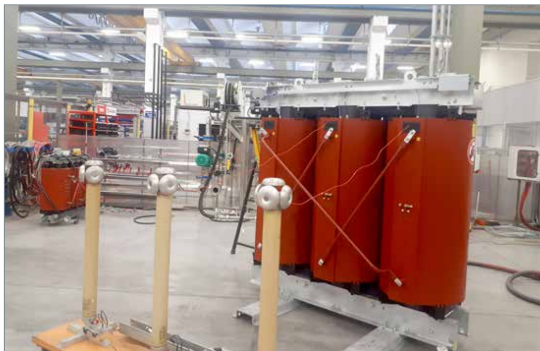
Measurement of partial discharge level during routine testing.
