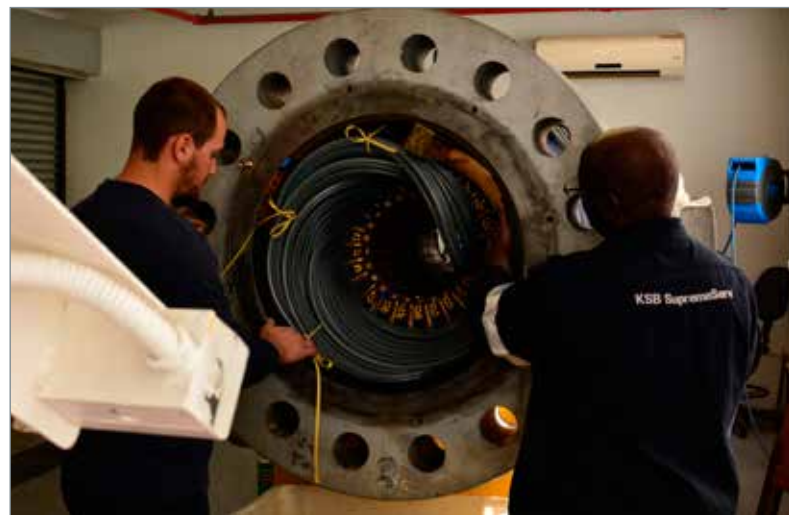
KSB Pumps and Valves technicians repairing a boiler circulating pump and motor.
