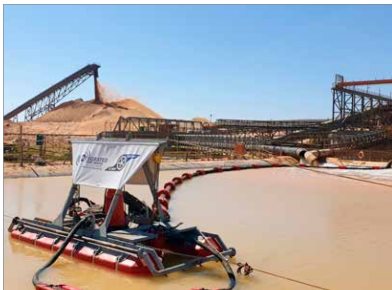
SlurrySucker dredging unit proved its value in a highly corrosive application.
