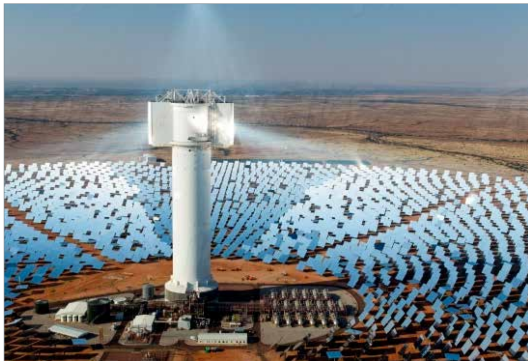
KHI Solar One plant near Uppington.
