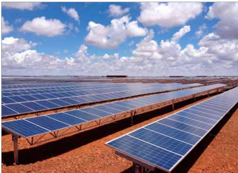
REISA Kathu Solar PV, Northern Cape.
