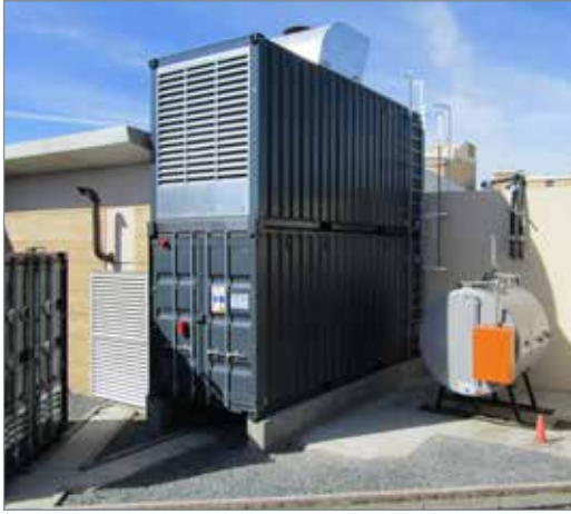
The genset installation provided by Zest WEG will expand the hospital's standby generating capacity to 1 MVA continuous rating, allowing 100% of the institution's functions to continue as normal during periods of load-shedding.
