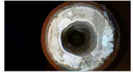
Photo shows 50mm pipe with scale measuring 10-12mm thick inside it. The flow of water has been dramatically reduced due to lack of maintaining the softener.
