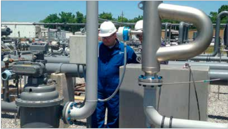
High precision: Promass Coriolis flowmeters enable high-precision measurement of a wide variety of liquids and gases as well as fluids with entrained gas bubbles.
