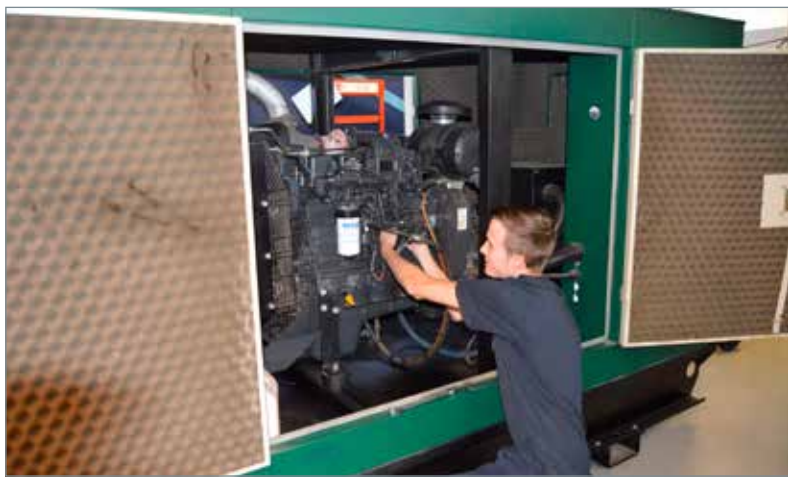
Specialist repairs on a generator diesel injection system underway at Reef Fuel Injection Services.
