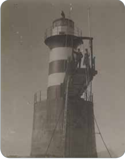
The lighthouse underwent several changes to its appearance, or daymark: originally, the lower half of the tower was painted black and the upper half white; between 1888 and 1902 the colour scheme was changed to red and white bands (as shown above); and on 15 November 1929 it was changed to all white with a red lantern house and dome. The lantern house and dome were later changed to white (TNPA Archives).
