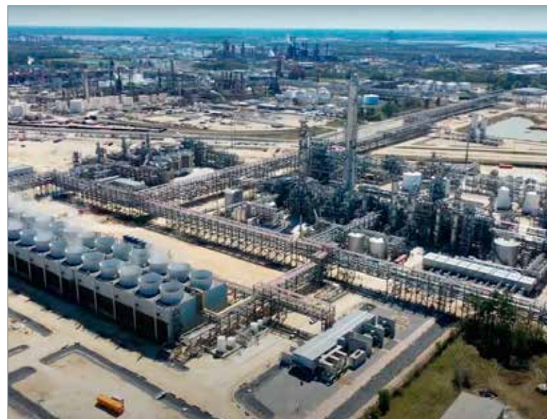
Sasol's Lake Charles troubled petrochemical facility.
