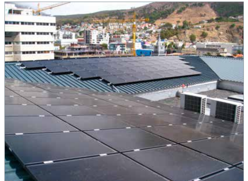
Cape Town is deploying rooftop solar plants to reduce the impact of load shedding.
