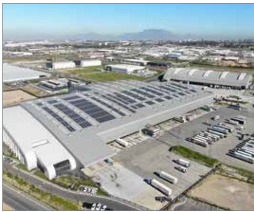
Solar panels at Shoprite's Basson distribution centre.
