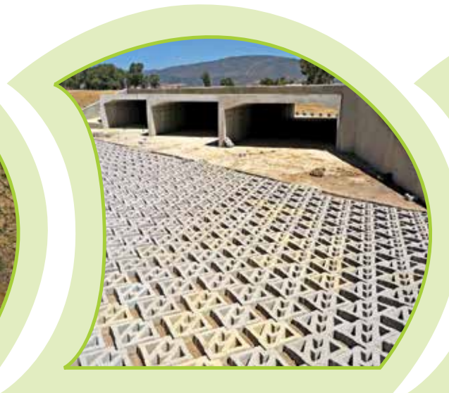
Terracrete permeable paver storm water management, Western Cape.
