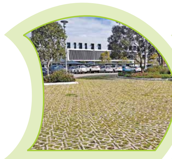
Grassed Terracrete parking, hospital, Western Cape.
