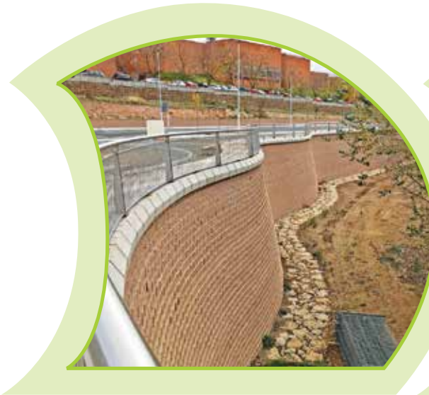
Beautifully curved near vertical Terraforce rock face wall, hospital, Spain.
