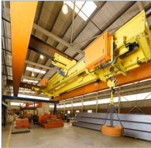
Condra telescopic crane under test.
