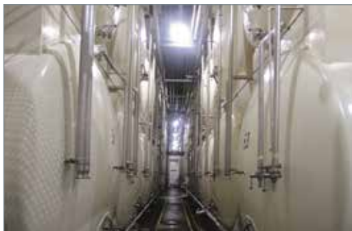
Application Keller Beer Tanks.
