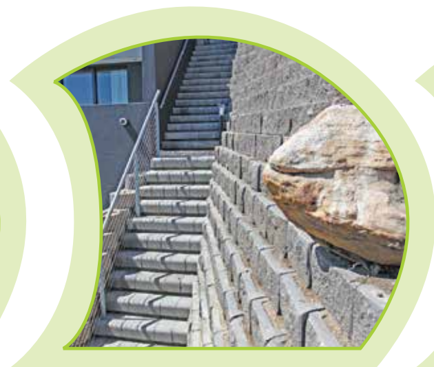
Stairs and rock-face retaining
