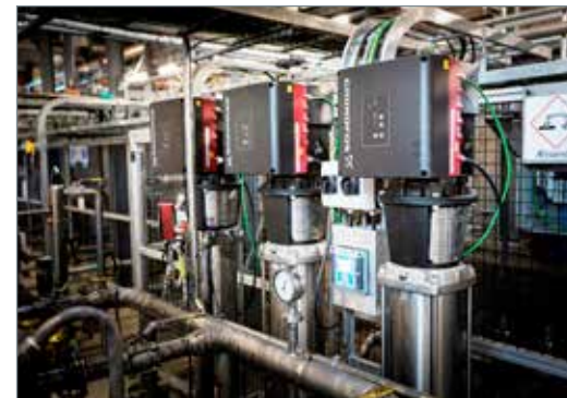
A Grundfos three pump booster set with cascade function; when flow varies across the plant the booster set can maintain constant pressure with varying flows depending on the wash and clean demand.
