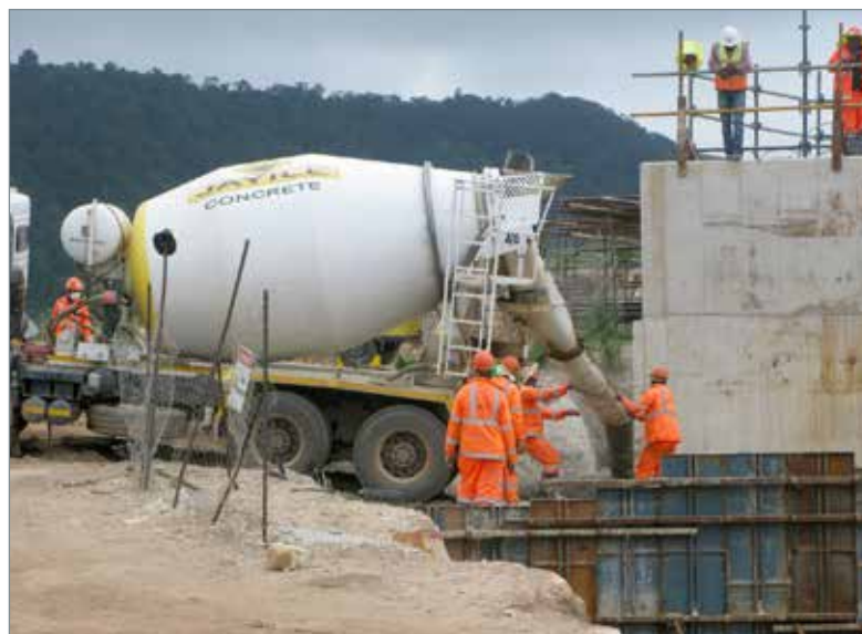
Readymix is being provided on the project by local SMME, Jayile Concrete. The aggregate stone is supplied and transported to site by local SMMEs sourced from a locally owned quarry.
