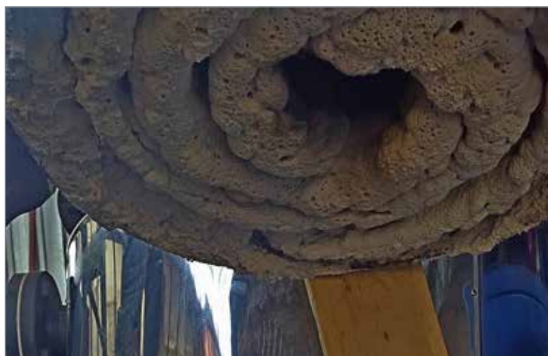
Electrode boiler head with excessive scale.
