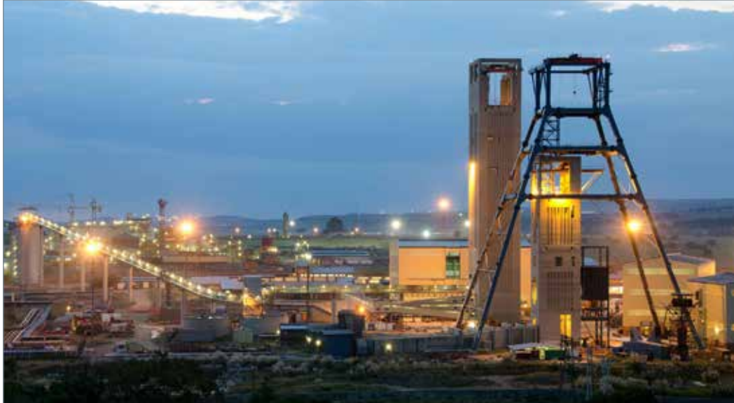
Goldfields South Deep Mine.
