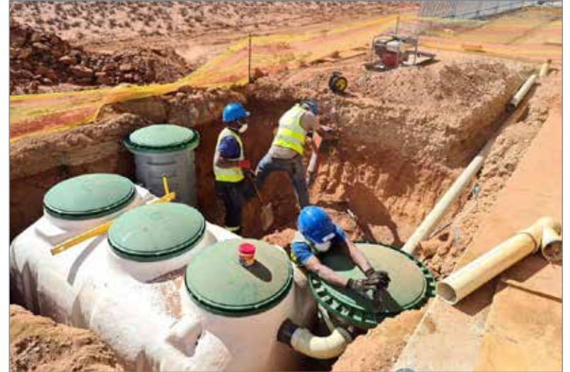
Installation of Clarus Fusion wastewater treatment plant.
