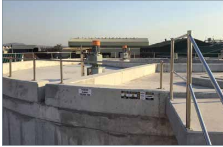
Nord sludge tank mixers.
