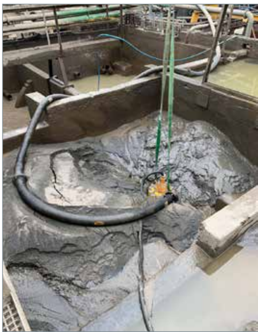
Goodwin 100ANZE submersible slurry pump - cleaning out a silted sump area.
