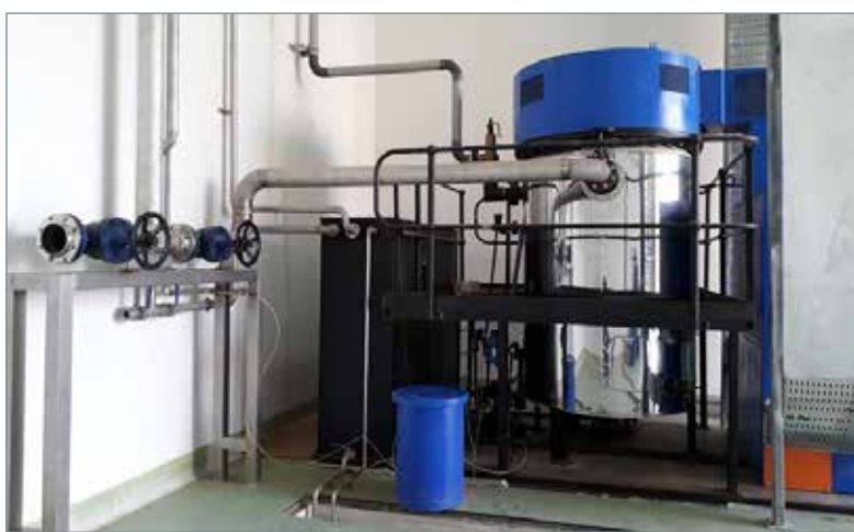
AA-2500 4 ton electrode steam boiler.
