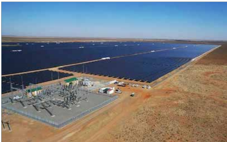
With double the output to the proposed Tharisa Mine project, the Paleisheuwel R82,5 MW solar project is a US$110 million (R1,750bn) utility-scale solar photovoltaic (PV) farm located in the town of Paleisheuwel, Western Cape. The solar farm consists of 611 000 panels and sits on 240 hectares of land.
