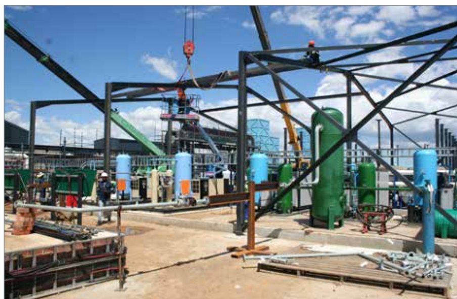
Renergen's cryogenic pilot plant during construction.
