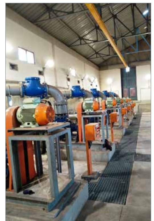
A return activated sludge pump station with power provided by WEG motors.
