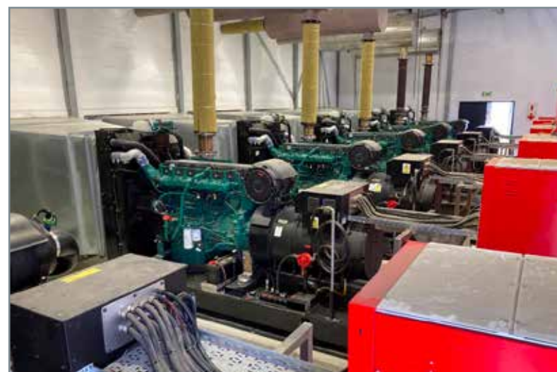
The 550 kVA gensets in the generator plant room on-site.
