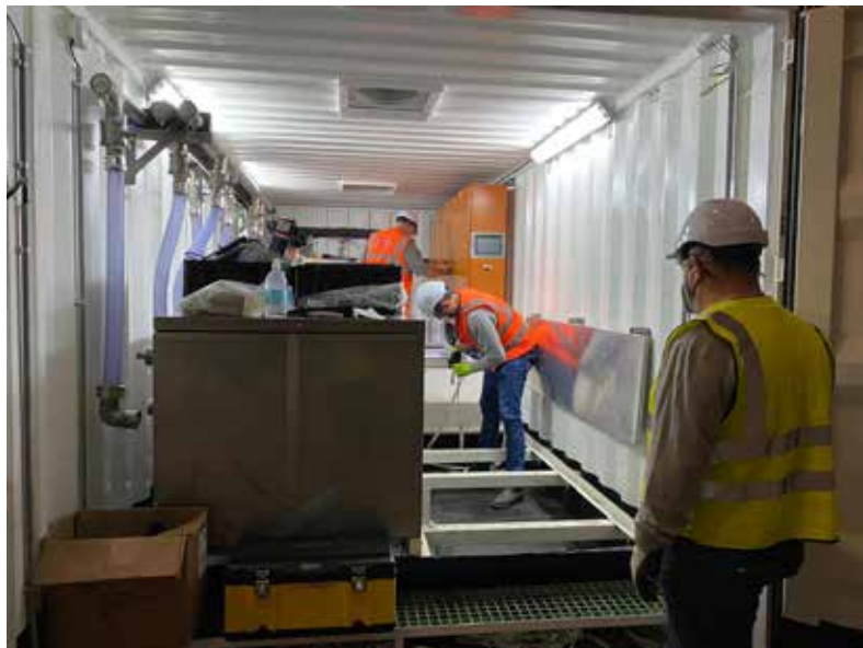
Fitting out the containerised plant.
