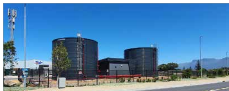
Typical SBS Tanks fire storage installation.
