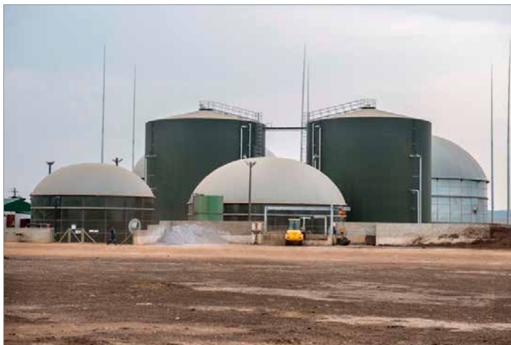
Bio2Watt's 4MW plant at Bronkhorstspuit, which supplies the BMW car plant in Rosslyn.
