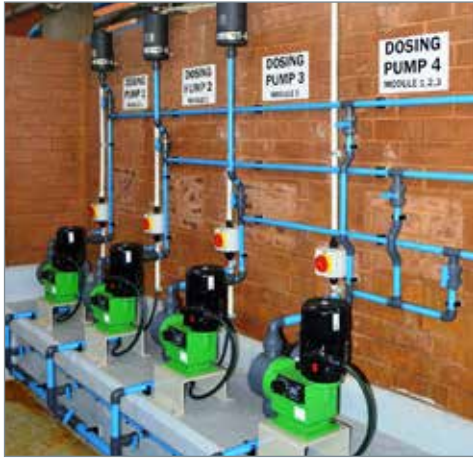
Grundfos DMX mechanical dosing pumps installed in a major municipal waste water treatment plants for dosing of Ferric Chloride.
