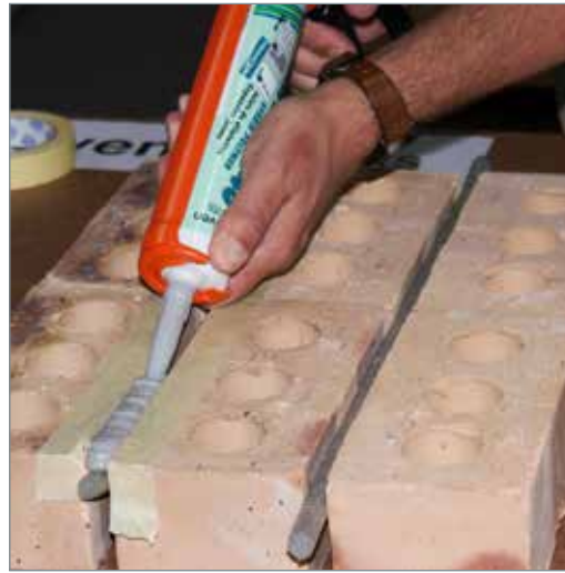
Demonstration using Hybriflex-540 with a backing cord for a three sided expansion joint and gap filling in brickwork.
