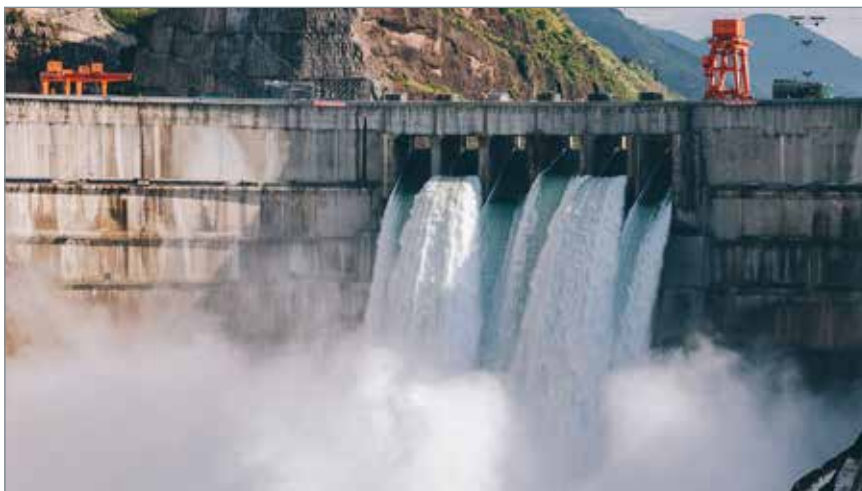
Gravity batteries work in a similar way to pumped hydro, which involves funnelling water uphill before releasing it through turbines to generate energy (Credit Getty Images)
