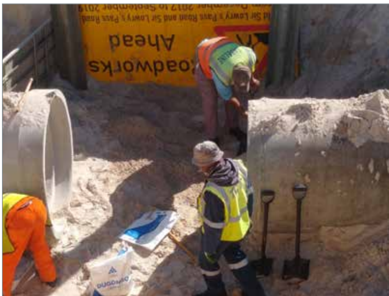
A manhole location during construction of the bulk stormwater pipeline, comprising approximately 300m of 1050mm diameter concrete pipes.
