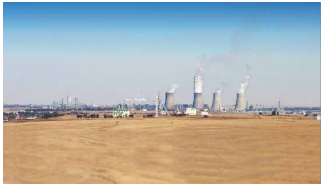
View across the Africa Energy – Sasol boundary, Sasol's Secunda plant.
