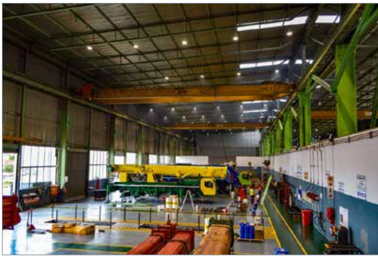
The locally designed and manufactured ECOBAY illuminates Liebherr-Africa's crane workshop
